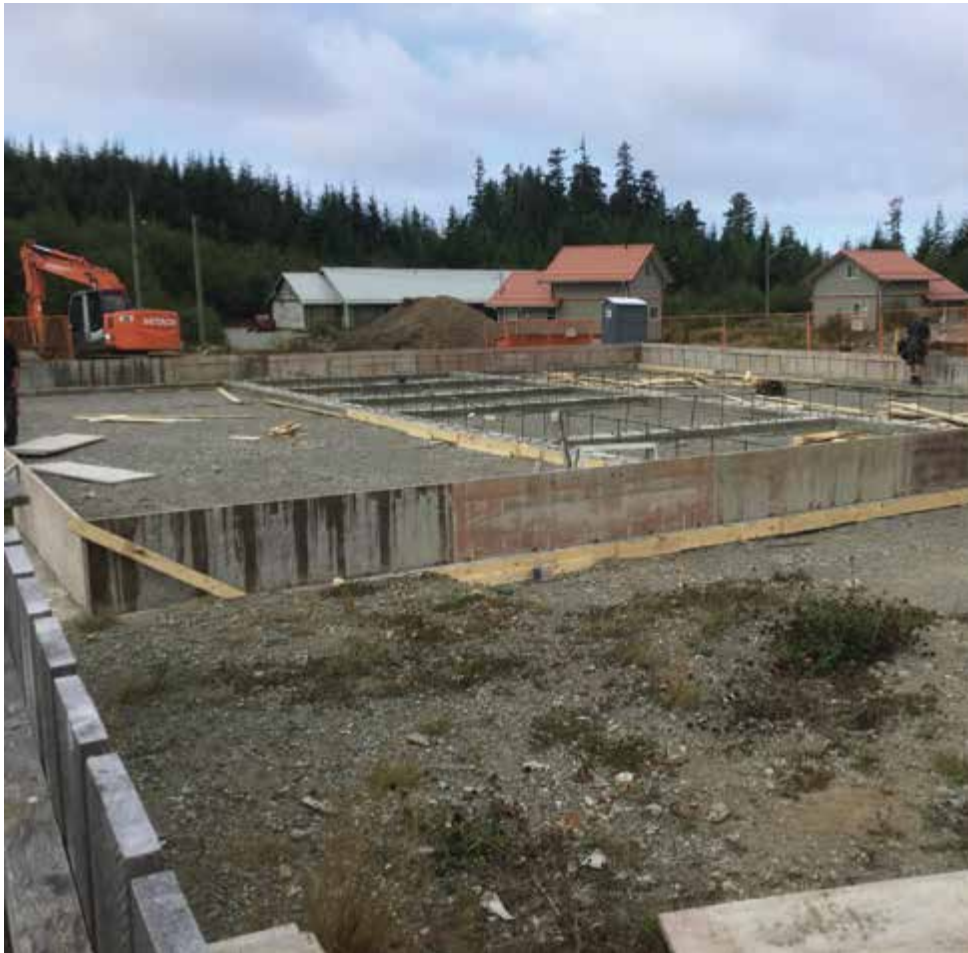
The foundation has been laid for the new Daycare building
